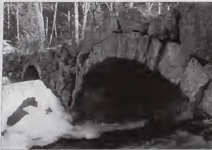
Above: The double-arched Carr Bridge in Hillsborough, New Hampshire, is a remarkable example of dry masonry stone work. A double-arched bridge allows for the necessary volume of water to flow through and still keeps the height of the bridge consistent with the roadbed. The granite was probably cut from deposits right by the river. Photo by Lynn Martin
